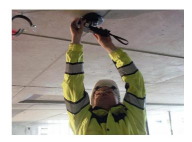
The readout of the data was done manually by a hand held reader. Alternatively, a fully automatic remote reading is available.
